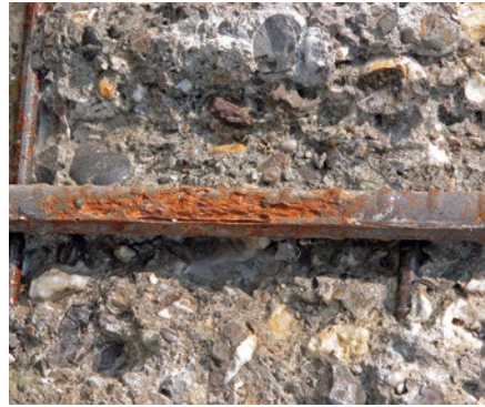
Fig. 8.2.1: Damage to concrete structure due to insufficient concrete cover and low concrete quality
