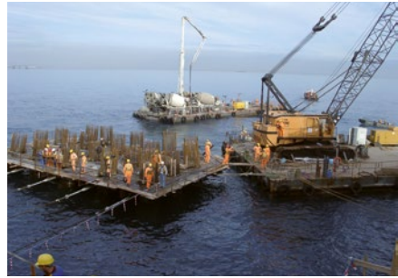
Fig. 8.14.1: When using underwater concrete, the placing and working conditions are very often complex, which is why these concretes often also need an extended working time.
